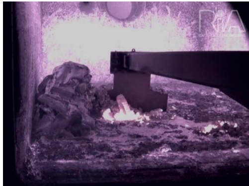
Figure 4. Levelling an uneven scrap pile.
